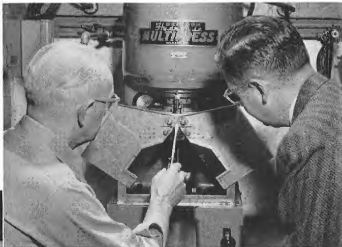
Roy Steinke slips a newly created guard into place, then shows its operation to Kenneth Pierson, Parker's safety director.
